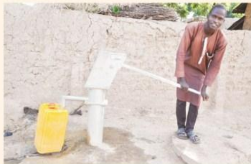
One of the numerous Hand Pumps constructed across the state
