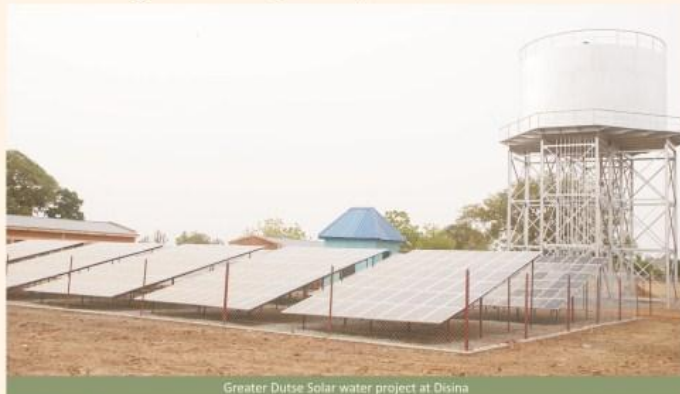
Greater Dutse Solar water project at Daina
